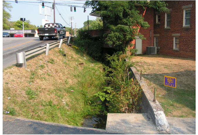
52 Tributary under Mill St. / 5th Street Intersection
