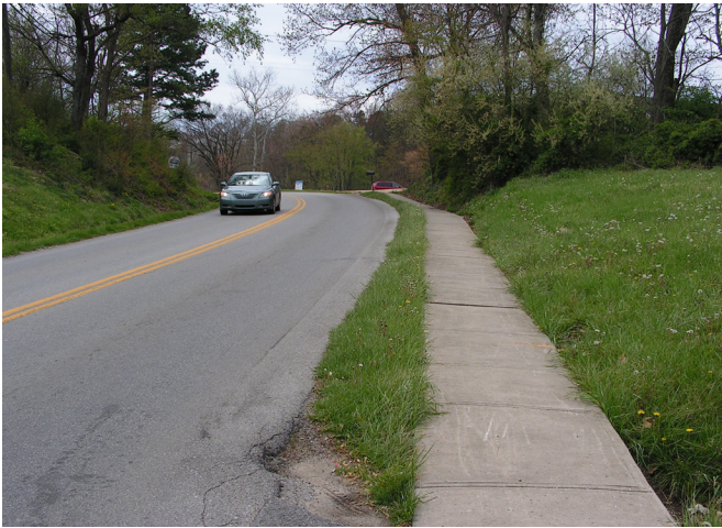
19 Between Stivers Lane and Greenway Drive
