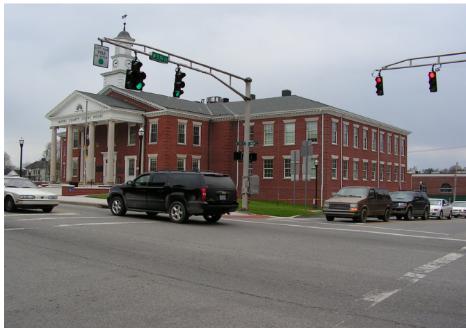
66 Laurel County Courthouse on US 25 at 5th Street
