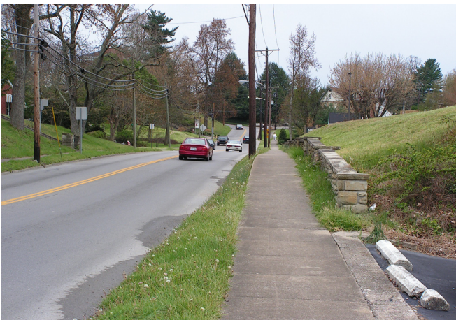
51 Old Stone Wall at St. William Catholic Church
